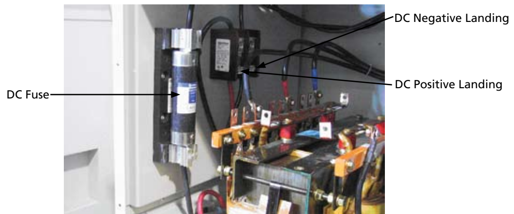
Figure 4-6 DC Wiring Procedure
