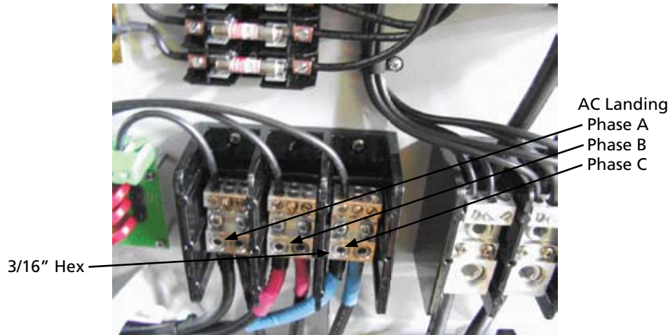
Figure 4-5 Inverter Connections
