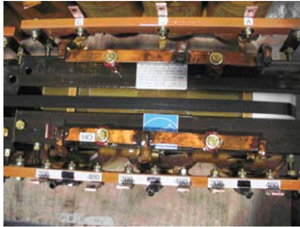
Figure 4-3 Tap Configuration
